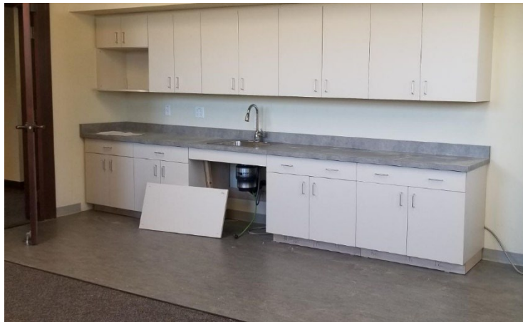
Ashland Staff Kitchen Renovation
